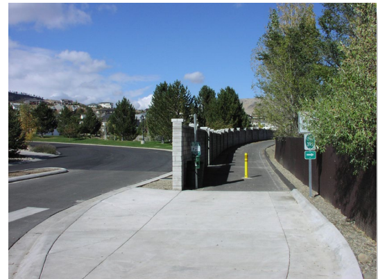
Desirable sidewalk conditions include: separation from traffic, shade and at least 5- to 6-foot wide.
