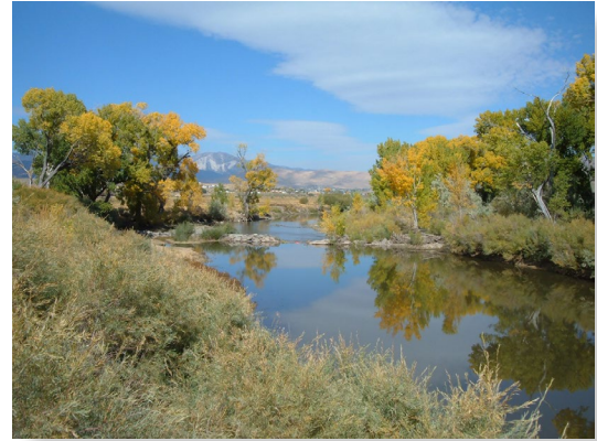
The Andersen Dam, a rockdam downstream of Carson River Road Bridge.
