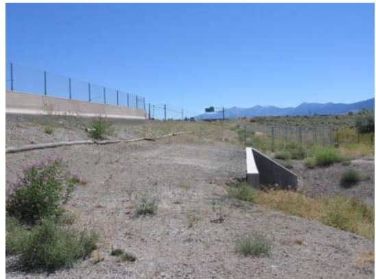
Looking south over the existing box culvert
