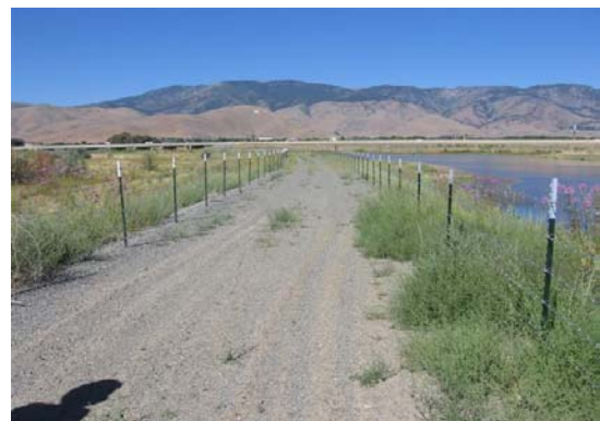
Maintenance road/weir between water quality basins and Kings Canyon Drainage
