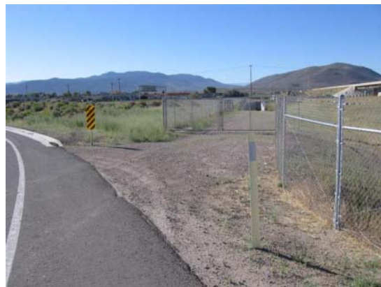
NDOT maintenance access
