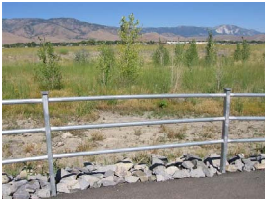
Typical railing at path drop-off
