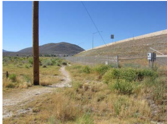
Looking south across Lompa property. Note existing use trail
